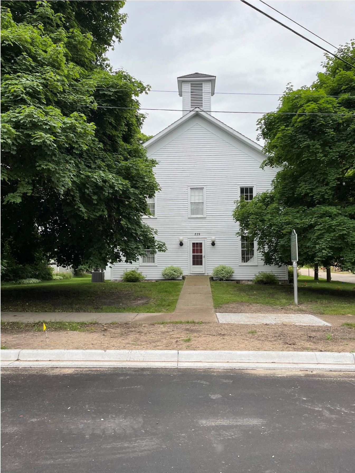
PHOTO C: The Building exterior after its restoration and as its current appearance.
