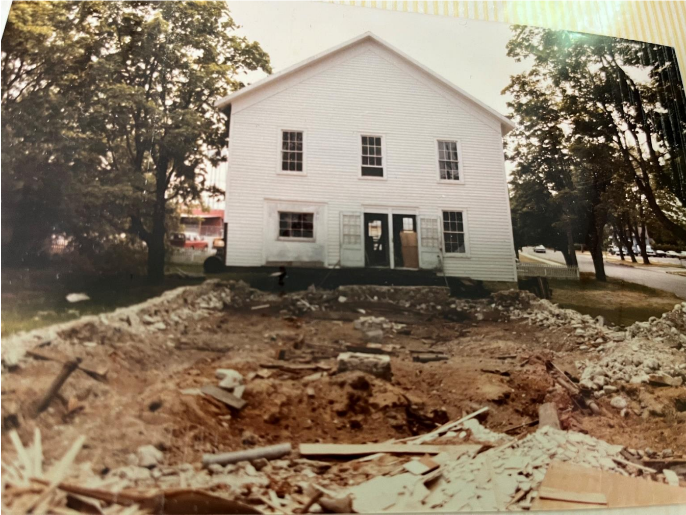
PHOTO B: The Building during its relocation.
