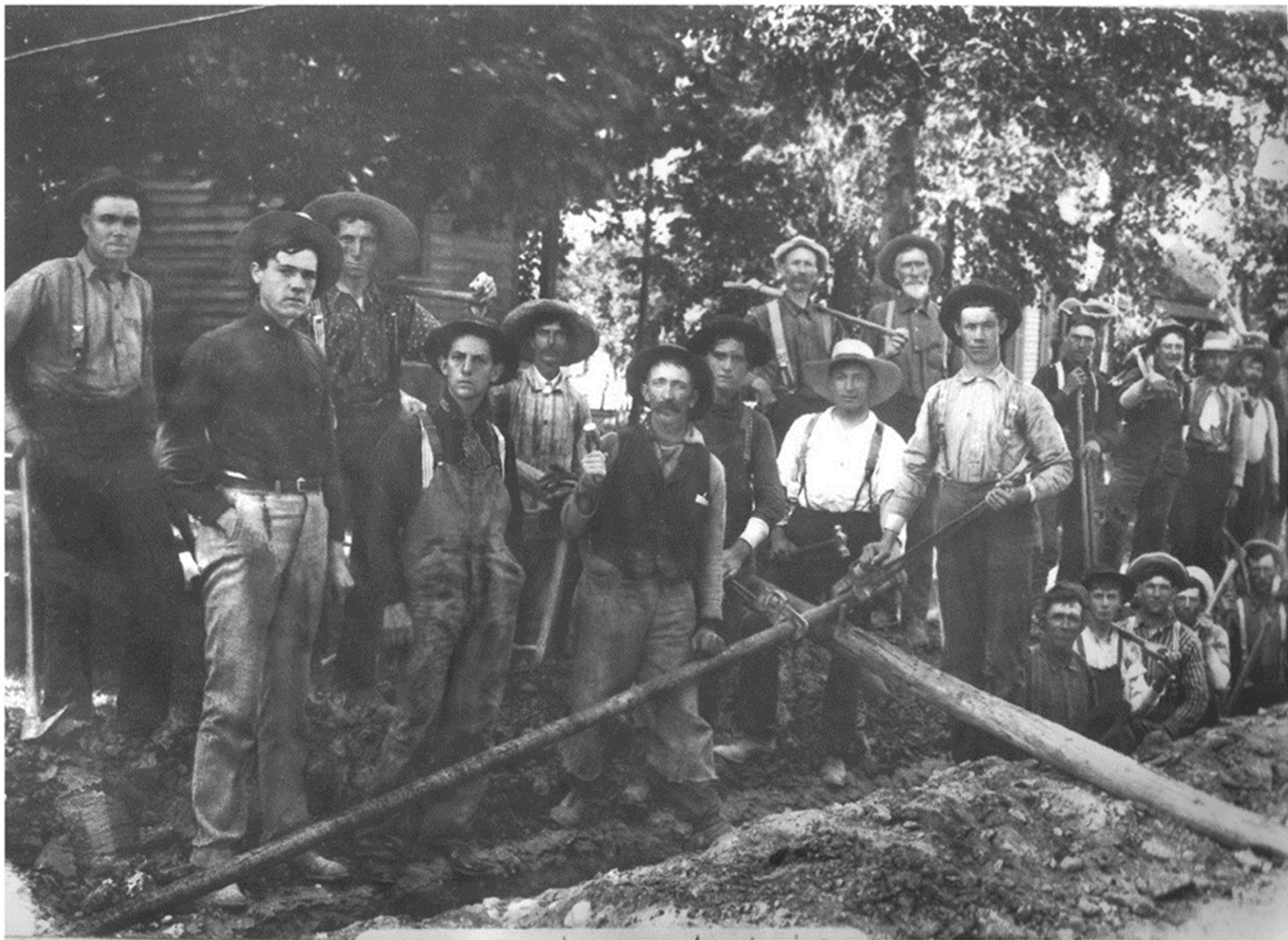
Laying Water Main - Cheboygan, Michigan
